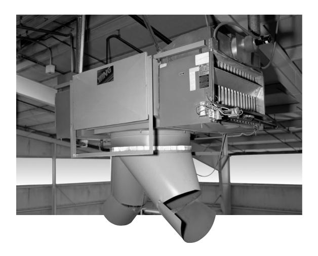
INDIRECT-FIRED GAS HEATING ASSEMBLIES FOR LARGE OPEN SPACES
